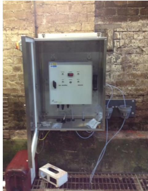
Unit installed in a wastewater plant in Scotland to detect high levels of VOCs
