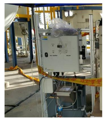
A picture of the unit installed in the outbuilding. The unit is connected to a PLC that records the data and, in case of an accident, triggers an alarm that switches off the intake pumps.
